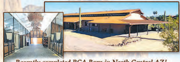
Recently completed RCA Barn in North Central AZ!
